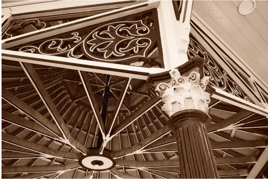
The Rotunda – Interior roof detail
