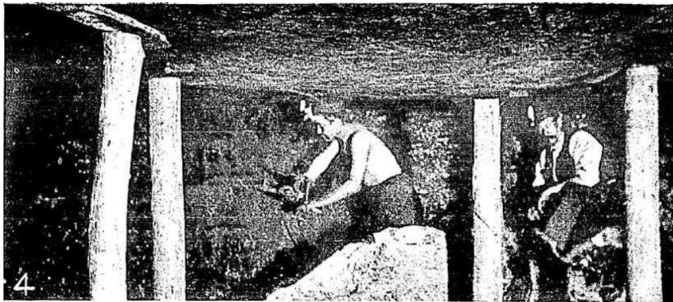
Boring a hole in the coal with a machine, Cooperative Colliery 1896 [2]
